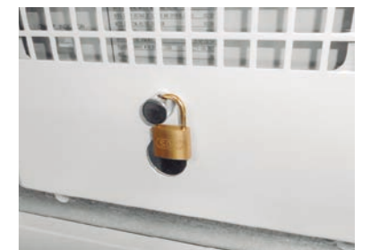
Fig. 3: Padlock for VCB operation
